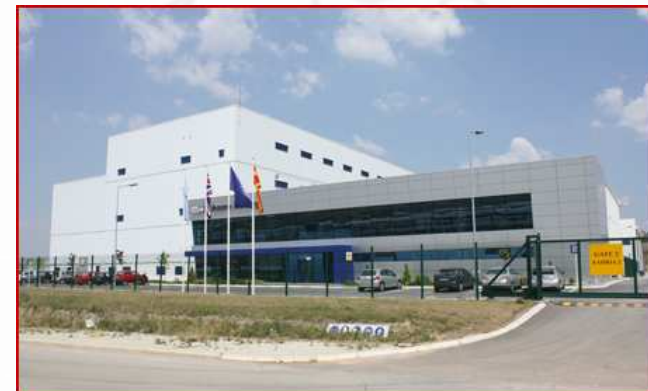
JOHNSON MATTHEY PLANT IN TIDZ SKOPJE 1
