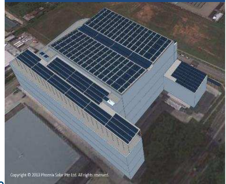
Singapore's largest PV system (1.4MWp) on Sheng Siong HQ,
